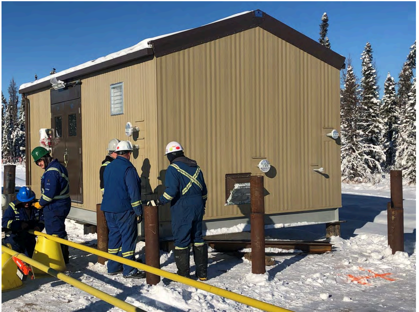
Figure 2: Installation New NGL Injection Skid
