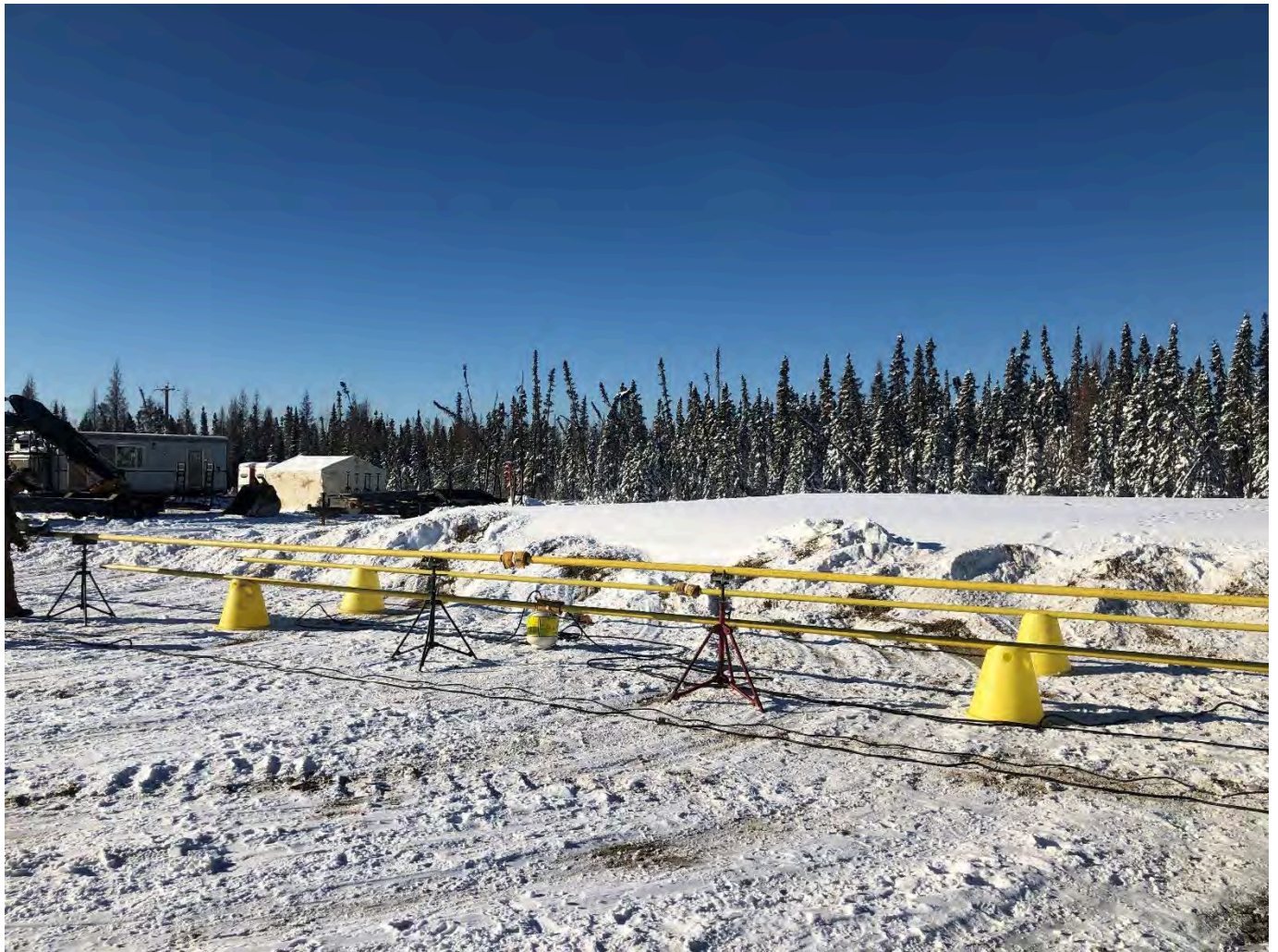
Figure 3: Preparing NGL' pipeline to connect Injection Skid to Injection Well
